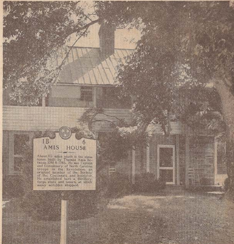
AMIS HOUSE , one of the historic landmarks of the Kingsport area, has probably changed little since it was constructed almost two centuries ago. It still contains some of the original furnishings which belonged to the first owner, Thomas Amis, great-great-grandfather of its present occupant. A highway marker erected by the Tennessee Historical Commission on Route 11-W between Kingsport and Rogersville marks the route to the stone house. (Times-News photos by Byland.)
